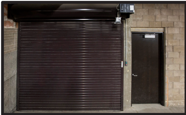
Loading Dock Door Size - 10' X 9'
